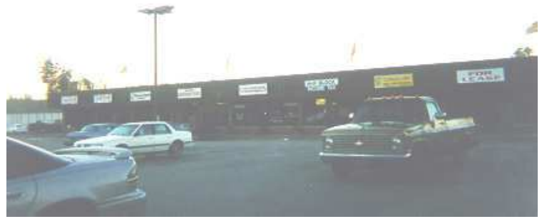
Figure C The Wadhams Plaza commercial development offers local residents a wide variety of services
